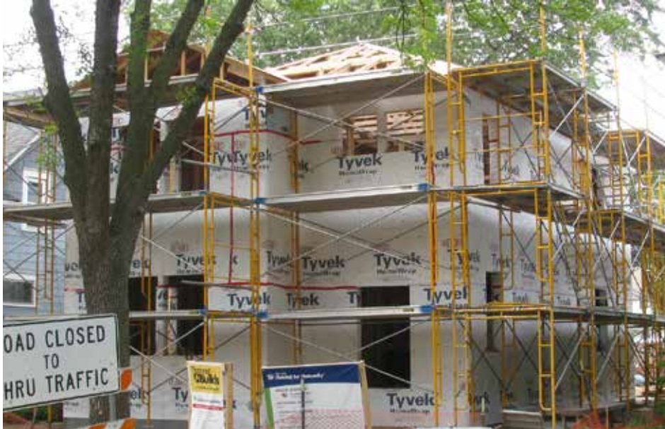
Faith Builders summer Habitat for Humanity home at 667 Lafond Avenue.
